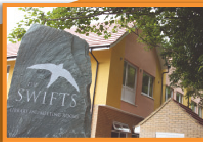
New meeting rooms and Library facility at The Swifts, Fulbourn.
